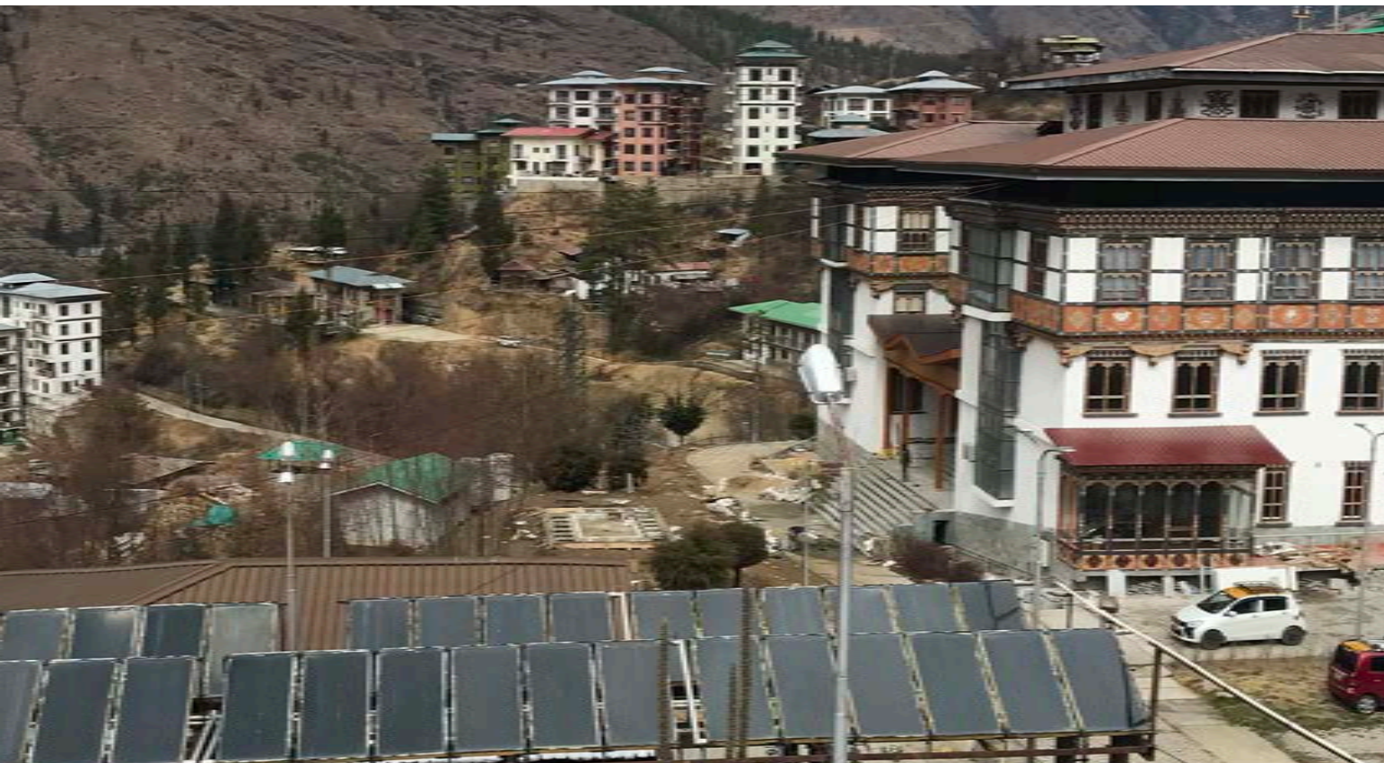
Figure 1.6 Thimphu IT Park and Solar Panels
