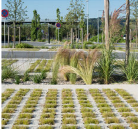
Permeable paving across parking areas
