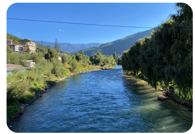
Enhancement of the river corridor | Source: TSP
