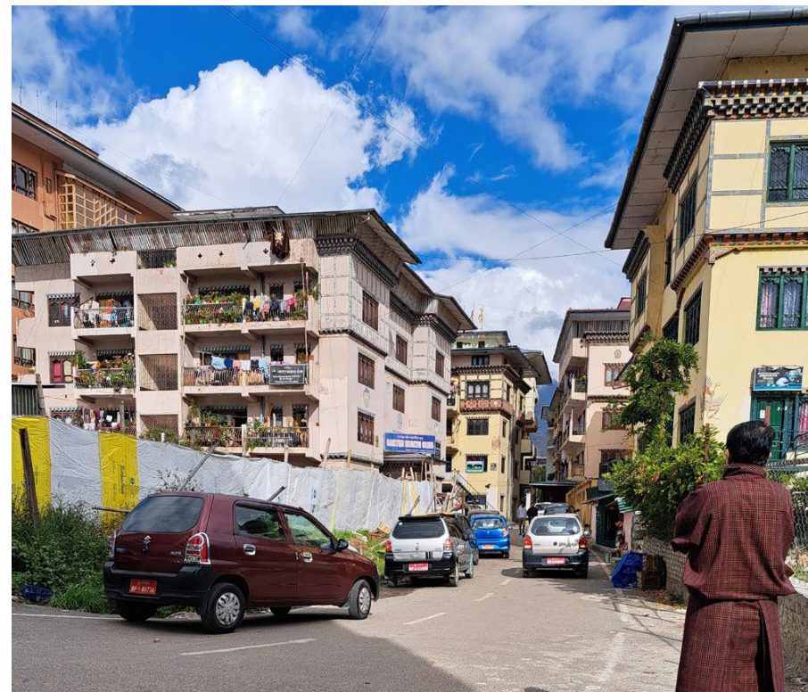
Lack of varied building typologies and no 'flex' according to specific use, context and any local character
