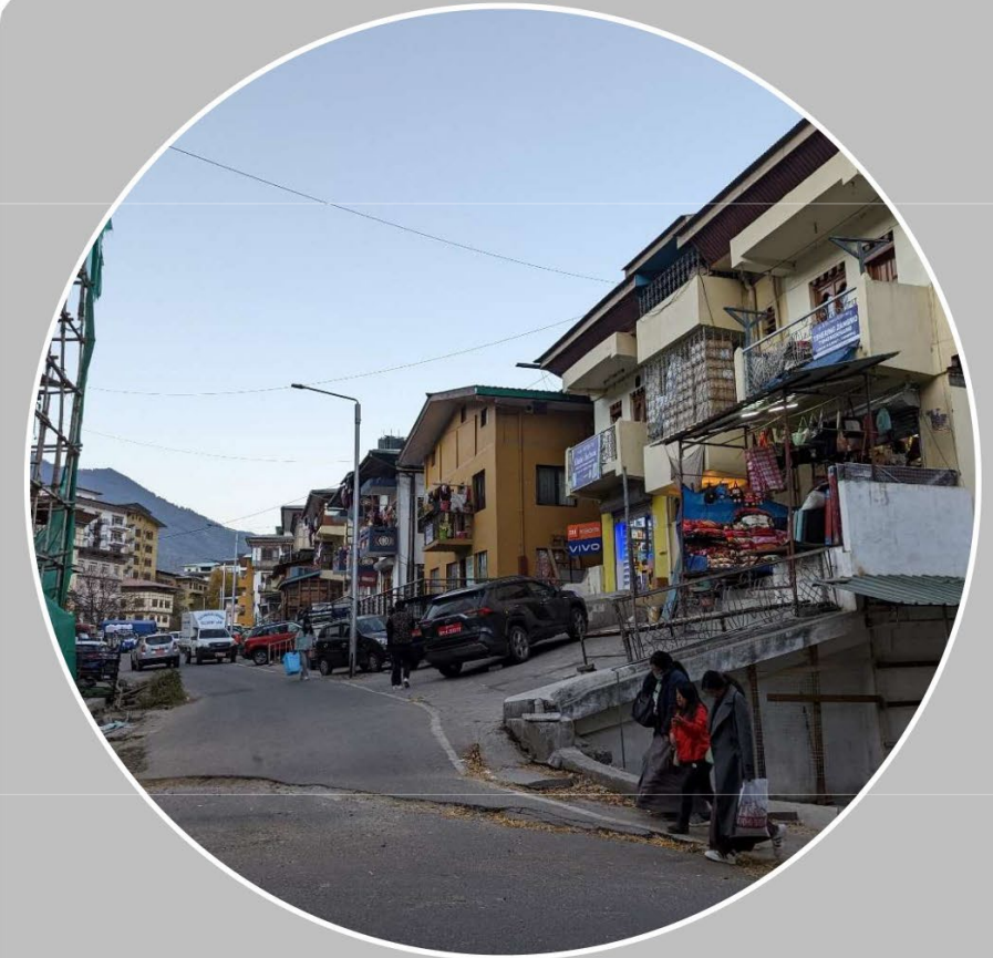
Improvement of existing road surface and paving
