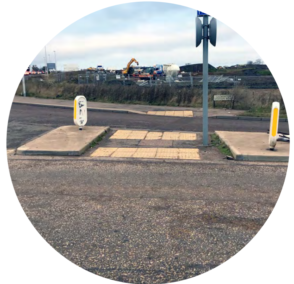
EXAMPLE SHOWS THE ACCESS TO THE LOANHEAD RAILWAY PATH.
