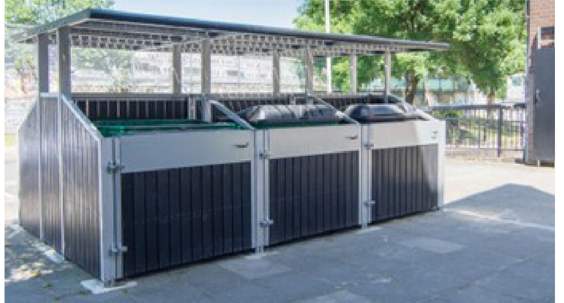
Figure 3.118 Segregated recycling bins for waste drop-off
