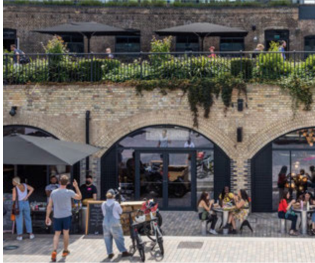
Figure 4.5 Coal Drops Yard, in London, a public square with activities at different levels.
