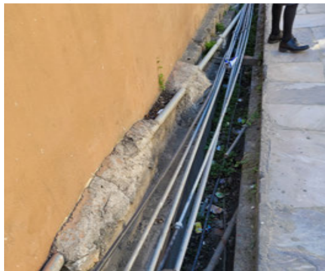
Figure 6.54 Utilities Laid in Stormwater Drain
