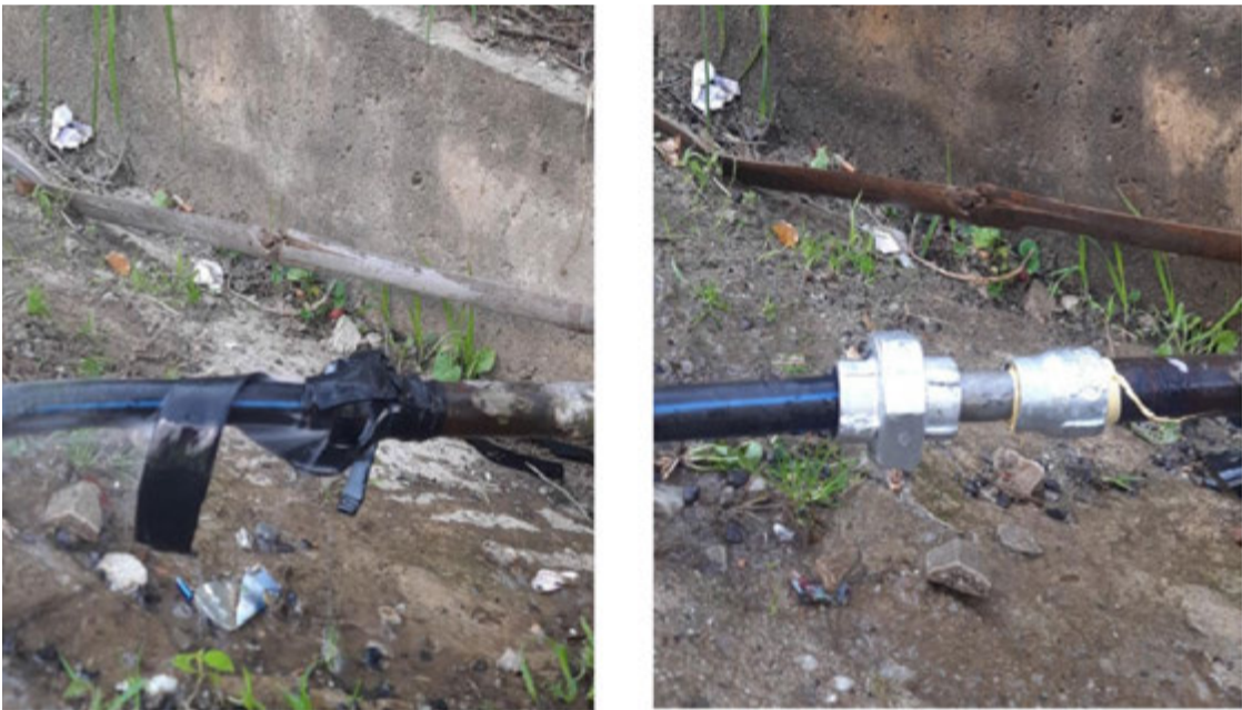
Figure 6.56 Leakage Repair Before/After (From Water Loss Audit)
