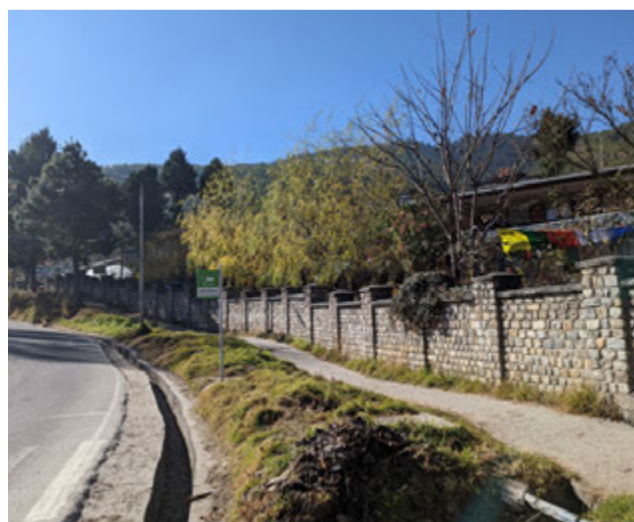
Figure 6.36 Disconnected bus stops from footpaths and the road
