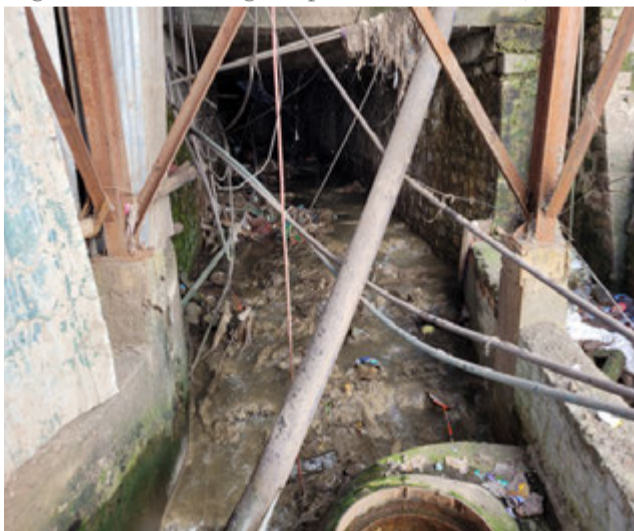
Figure 6.51 Existing Stormwater Culvert
