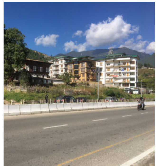
Figure 3.34 Doebum Lam - existing frontage and condition
