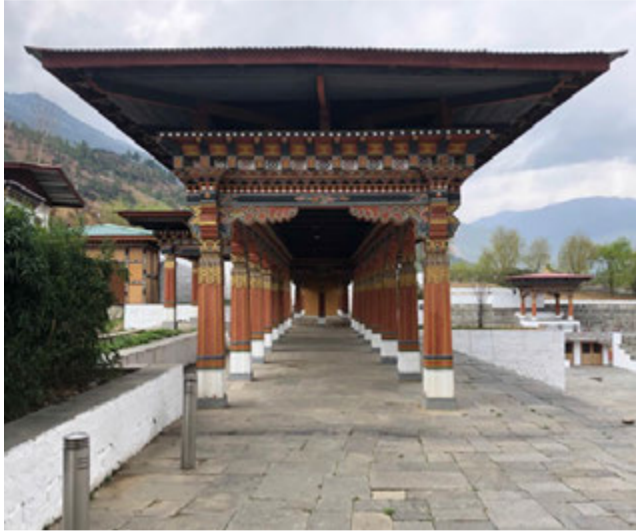
Figure 4.7 Pavilion in the Tashichho Dzong helping frame and enclose public spaces, while providing shade and shelter during events.
