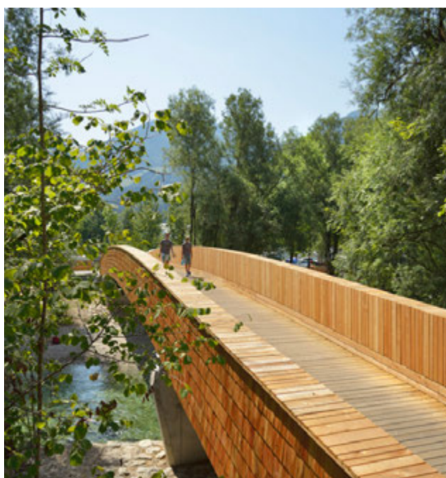
Figure 3.91 Pedestrian footbridge in Bohinj (SI)
