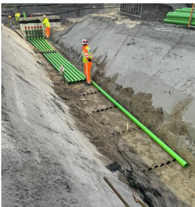
Figure 3.114 Duct installations and London Olympic Park
