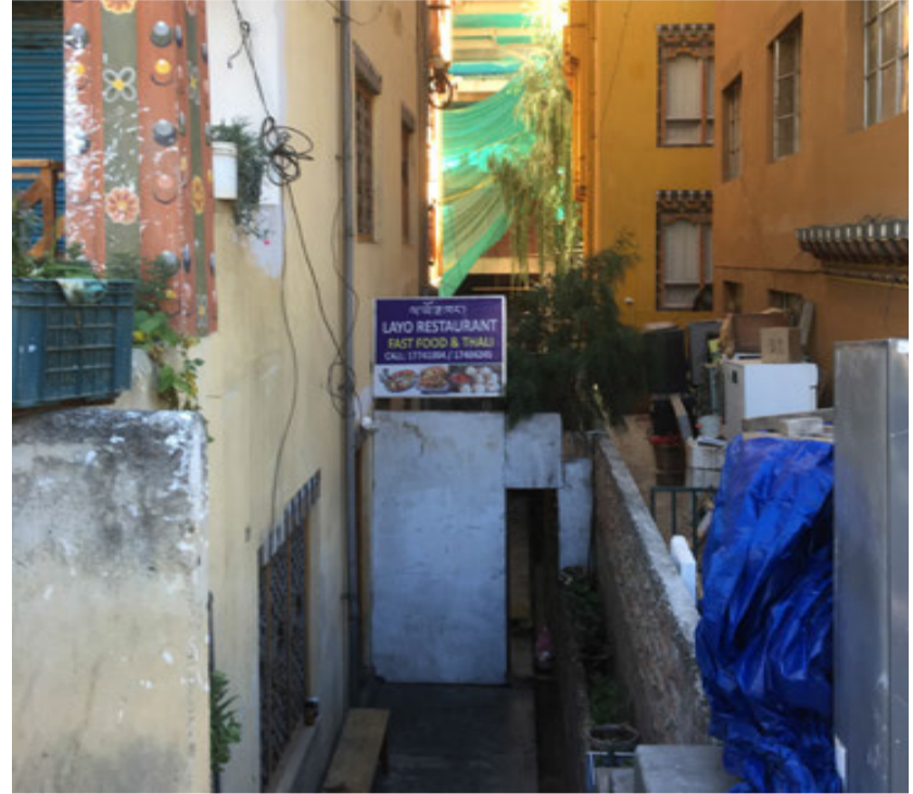
Figure 6.10 Lack of spaces between buildings for gathering areas
