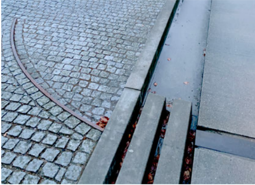
Figure 4.31 Incorporation of SuDS in narrower streets could be through open channels and rills
