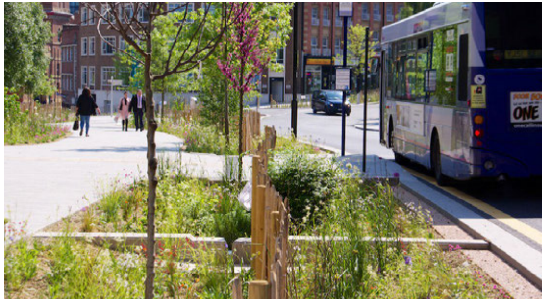
Figure 4.41 Sheffield's 'Gray to Green' scheme demonstrating how spaces for pedestrians, SuDS and buses could be organised along Chang Lam.
