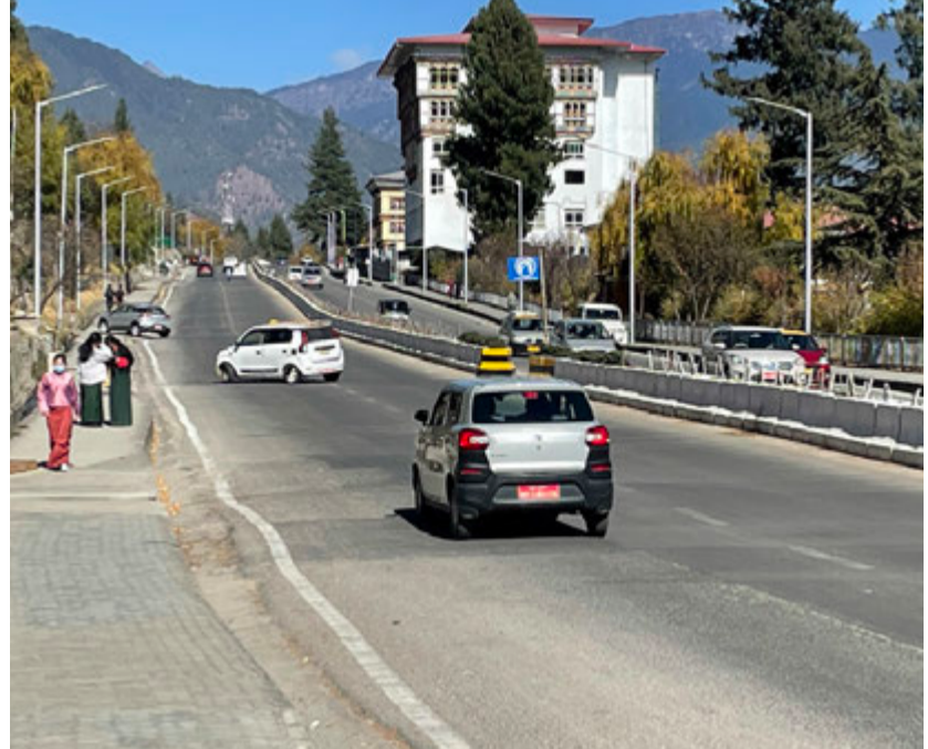
Figure 6.38 U-turn locations on the Expressway result in unsafe traffic conditions.
