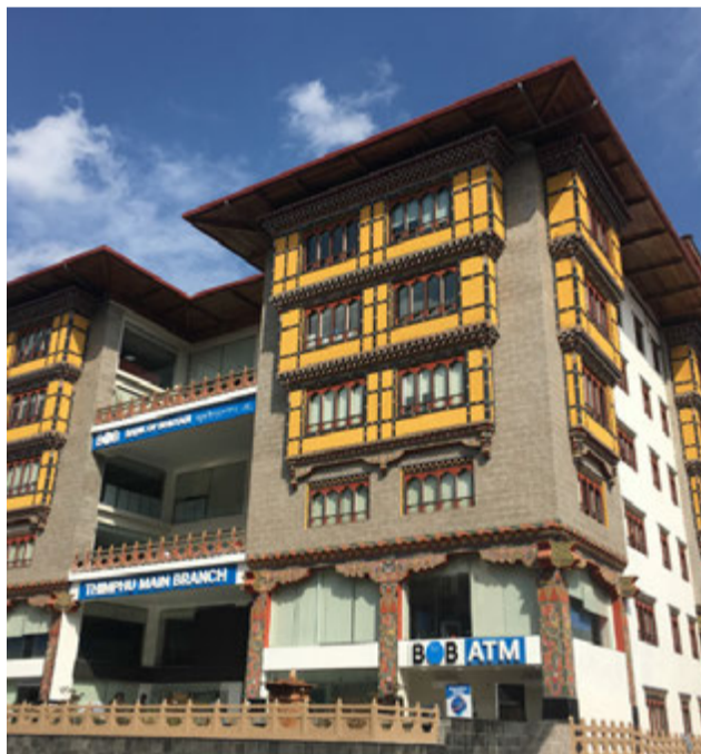
Figure 3.15 Existing- Bank of Bhutan
