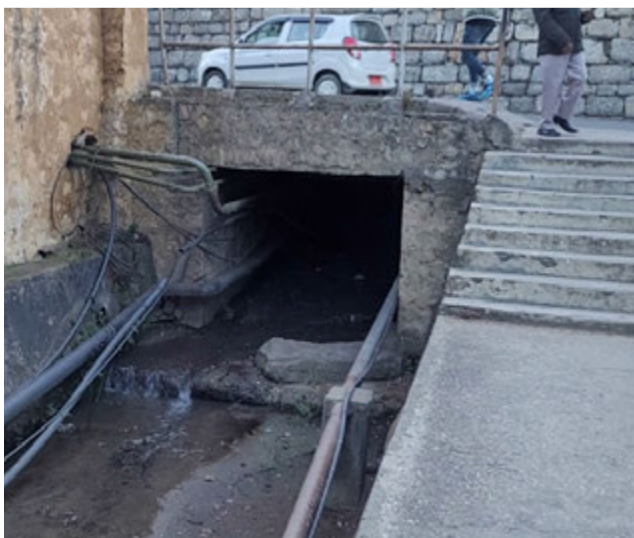
Figure 6.52 Utilities laid through Stormwater Culvert
