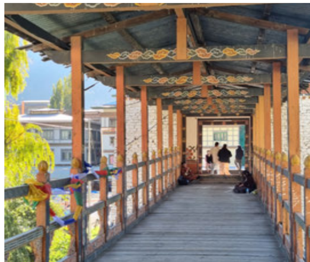
Figure 6.68 Wangchhu traditional bridge connecting Kaja Throm to the Riverside Crafts Market
