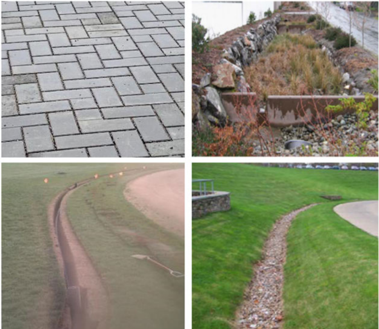
Figure 6-4: Examples of Additional SuDS depicted Clockwise from Top Left: Permeable/Porous Pavement; Perforated Lateral Drain; Swale; and Filter Trench
