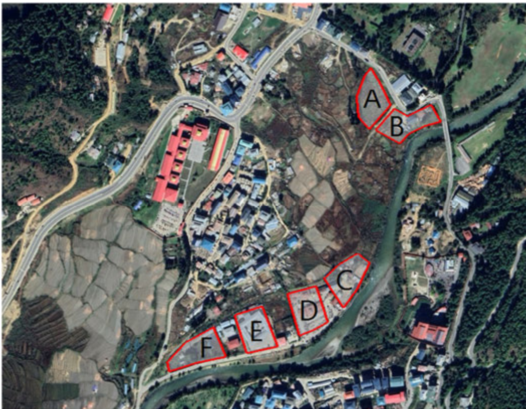
Figure 5-11: Location Assessed for the New Hejo WWTP
