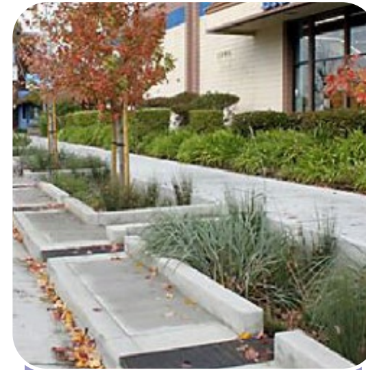
Sidewalkrain gardens - Example of sustainable Drainage System
