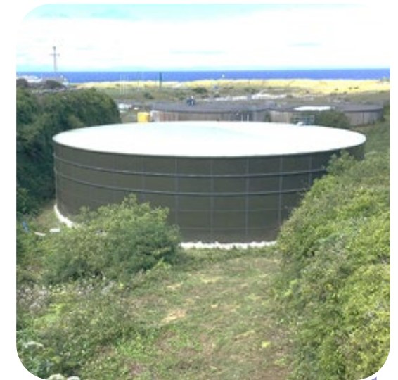
Raw water storage tanks - Example of sustainable Drainage System
